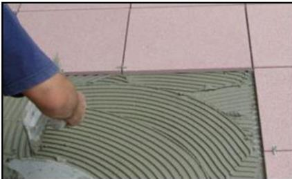
Figure 24 : Application Colle – Mortier/colle
